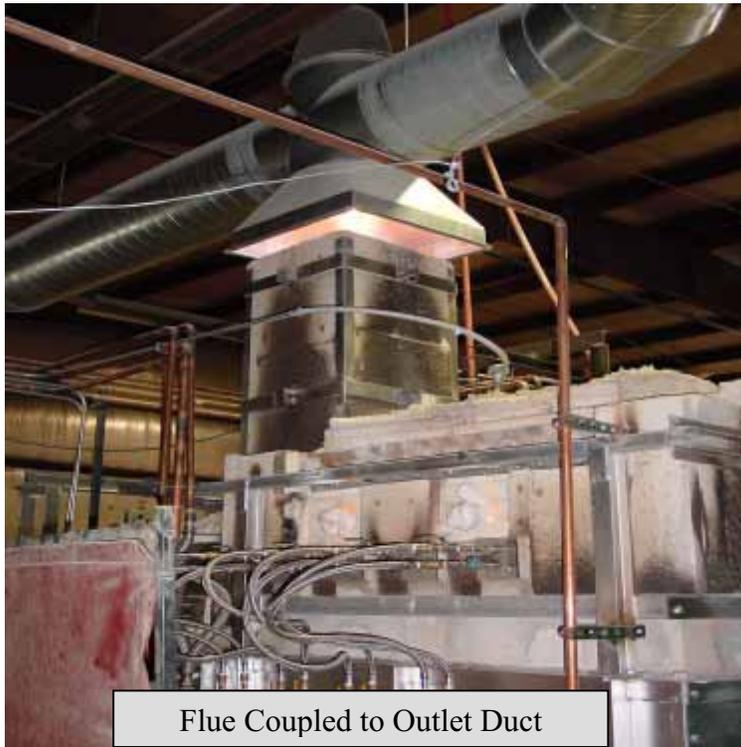
Flue Coupled to Outlet Duct
