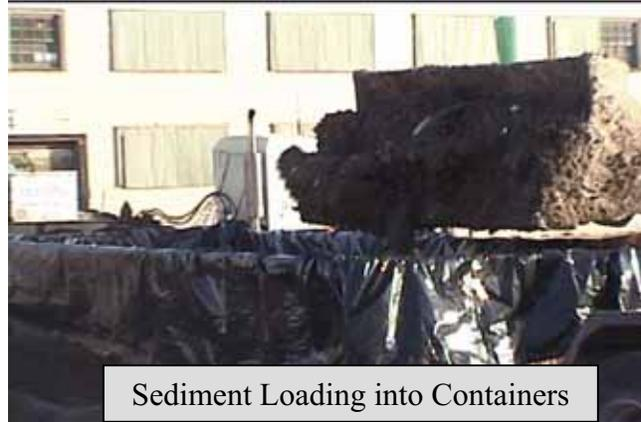
The U.S. EPA Superfund Innovative Technology Evaluation (SITE) program was used to perform an independent evaluation of the fate of PCB and other contaminants for Phase III. The dryer segment of the analysis was performed at the Hazen Research, Inc. facility in Golden, Colorado in January 2001. At that location, Hazen has a demonstration-scale dryer of the appropriate technology for use on sediments.
